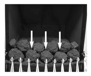
e) Select five of the large coals and arrange along the rear of the fuelbed, using the ribs in the rear of the fuelbed as a guide for placement. (See fig. 17 below)
