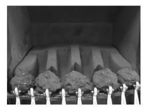
d) Select four of the large coals and arrange behind the front row of coals, ensuring that flame paths as indicated below are not interupted. Select two of the small coals and place at each end of the second row
